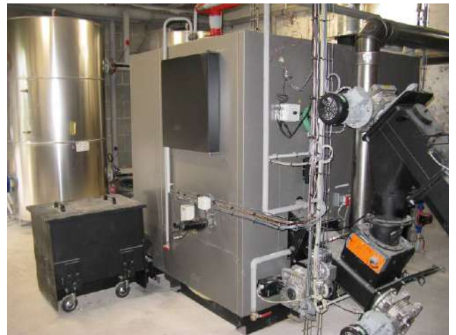
Chaudière FRÖLING Turbomat 220 kW
